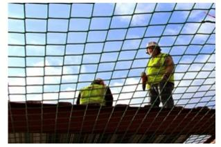
The number of workers protected by an individual Safety Net that complies with BS EN 1263-1 & 2, must be contained within the capacity of the net. Therefore, for a 2m maximum fall height, and allowing 100kg per worker including tools, this would set the recommended maximum number of 2 workers over any section of Safety Net.
