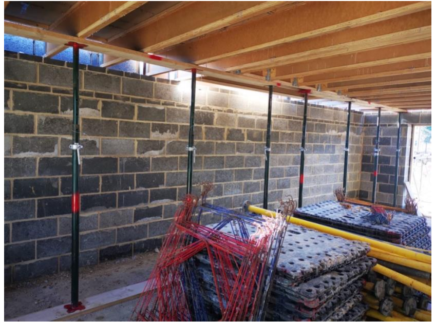
Figure 1. Example of Back Propping.
